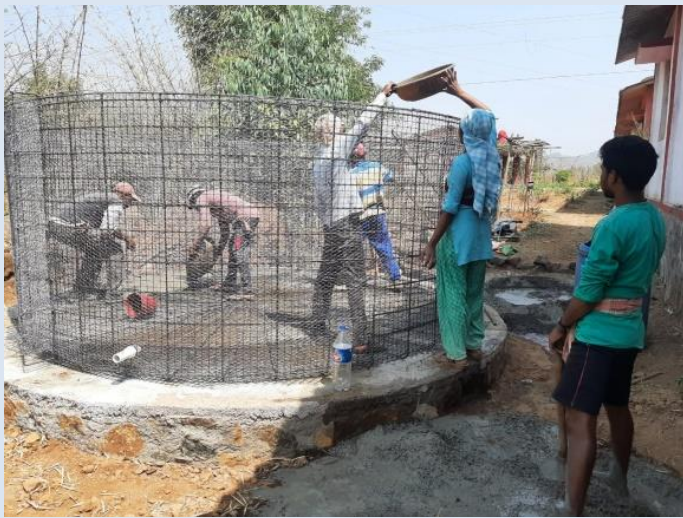
Ferrocement Tank Under Construction
