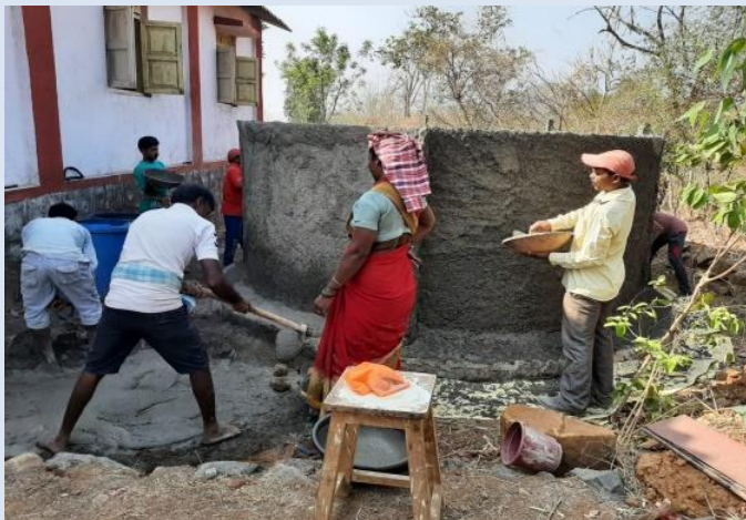
Ferrocement Tank Under Construction
