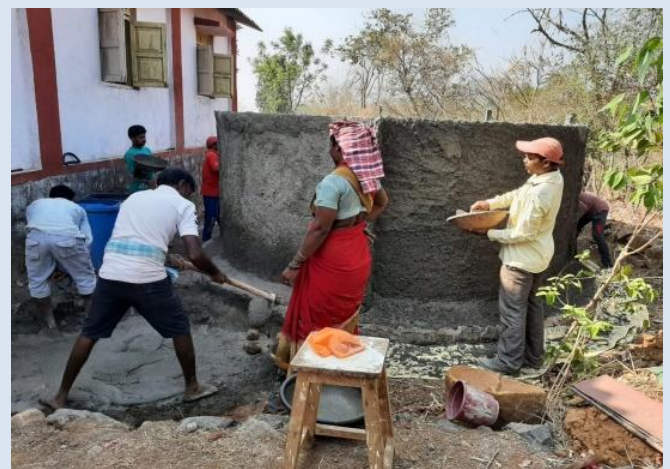
Ferrocement Tank Under Construction
