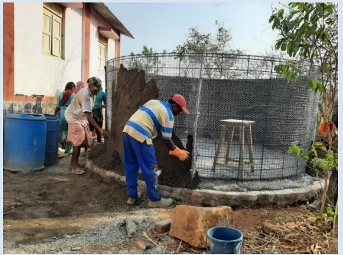
Ferrocement Tank Under Construction
