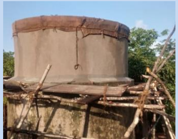
16. Ferrocement Tank at Sade wadi 10 feet in dia and 4 feet in Height Krishna Utekar by Local Mason in September----- P 10
