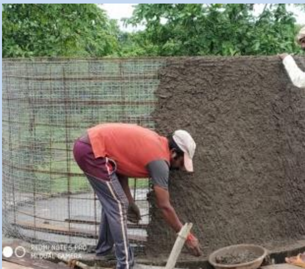
16. Ferrocement Tank at Sade wadi 10 feet in dia and 4 feet in Height Krishna Utekar by Local Mason in September----- P 10
