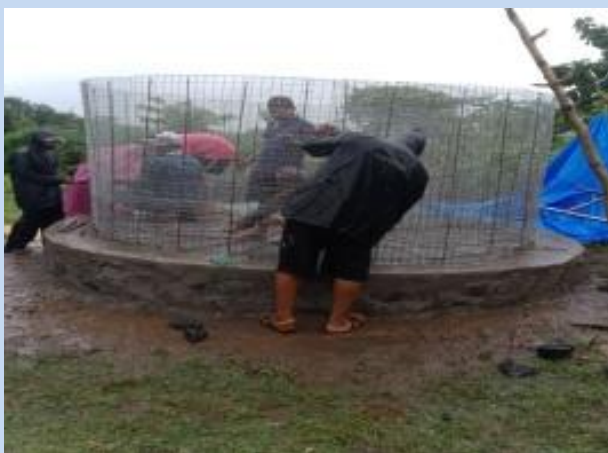
19. Ferrocement Tank at Anvir ,Thakarpada, Taluka Talasari for Yashraj Foundation 13th to 17th September ----- ----- SC--- 4
