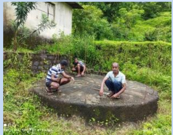
16. Ferrocement Tank at Sade wadi 10 feet in dia and 4 feet in Height Krishna Utekar by Local Mason in September----- P 10
